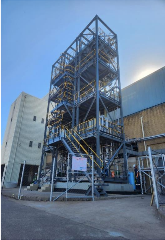
Figure 1. Crystallizers at the Demo Plant
