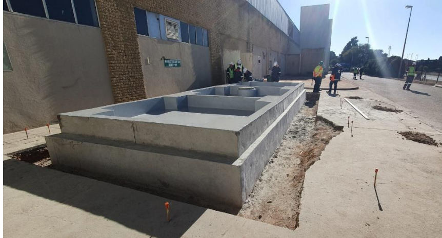
Figure 3 Prepared crystallizer unit foundations.
