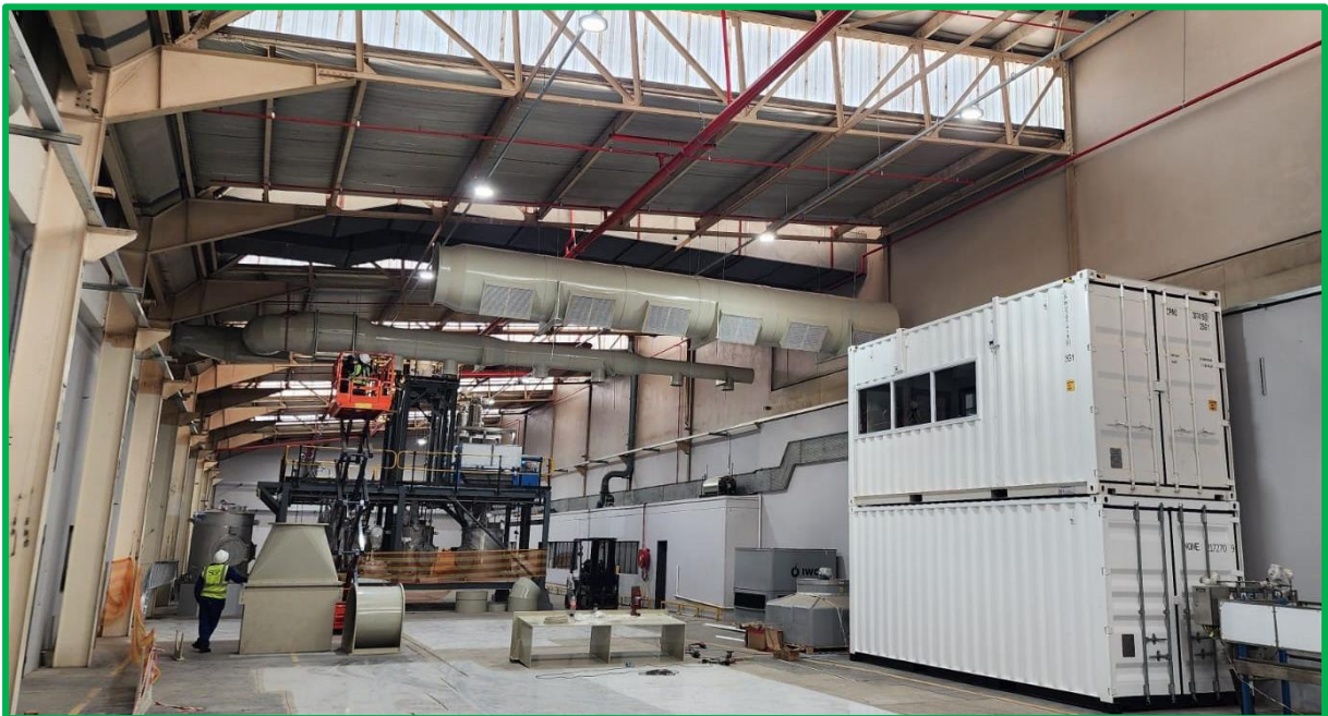
Figure 4: Installation of Control Room Units and Preparation for Next Process Modules
