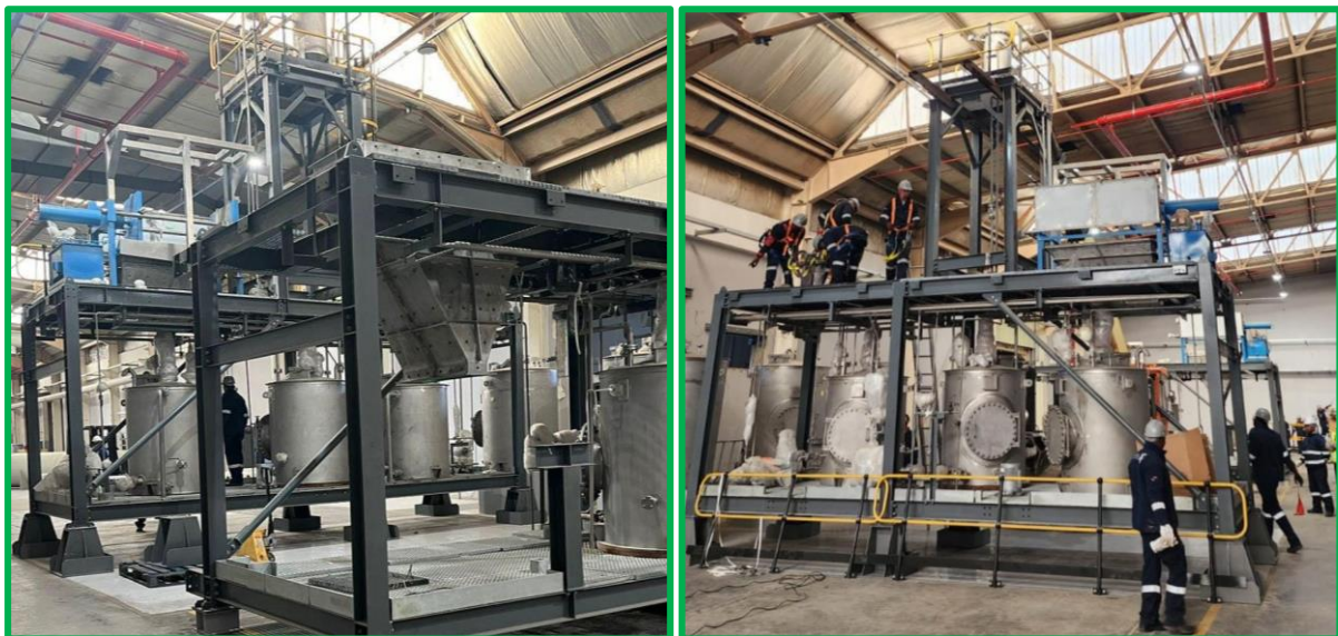
Figure 1: The First Two Process Modules are now in Place
